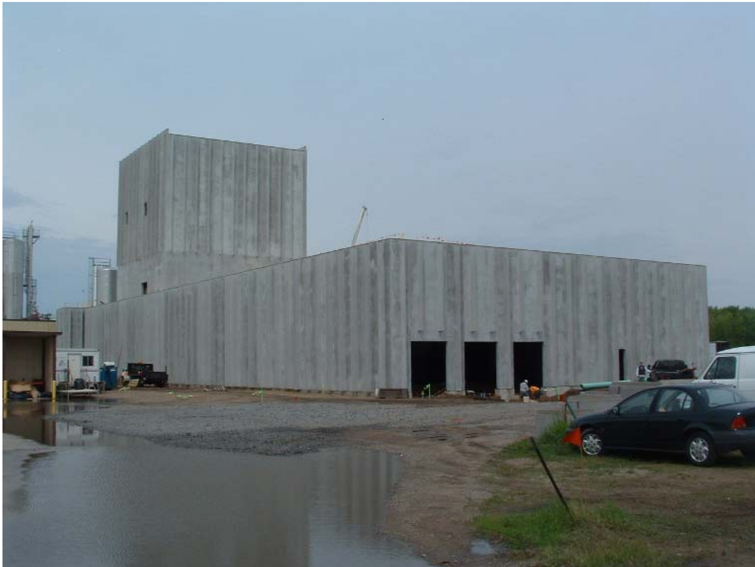
Drying Tower & Warehouse
